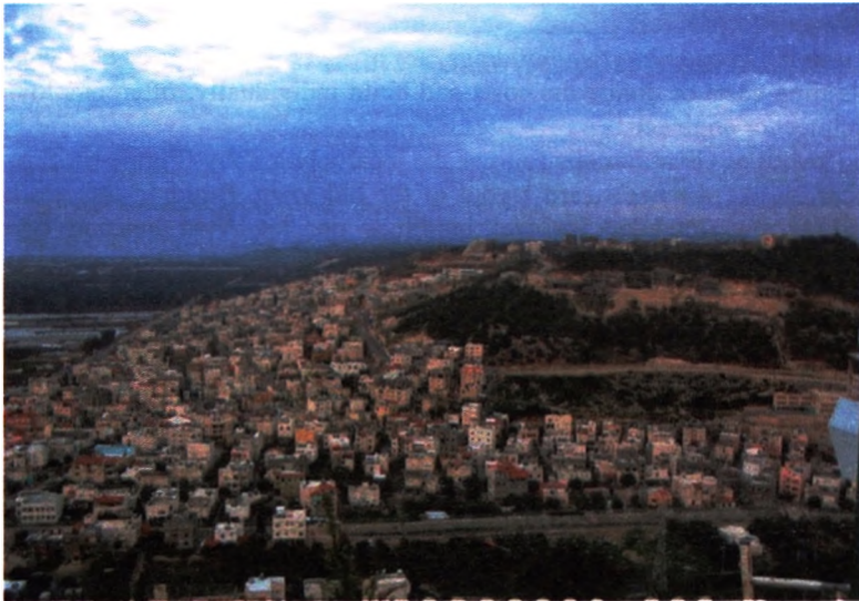
Figure 5: Givat Faradis, under construction above Faradis
