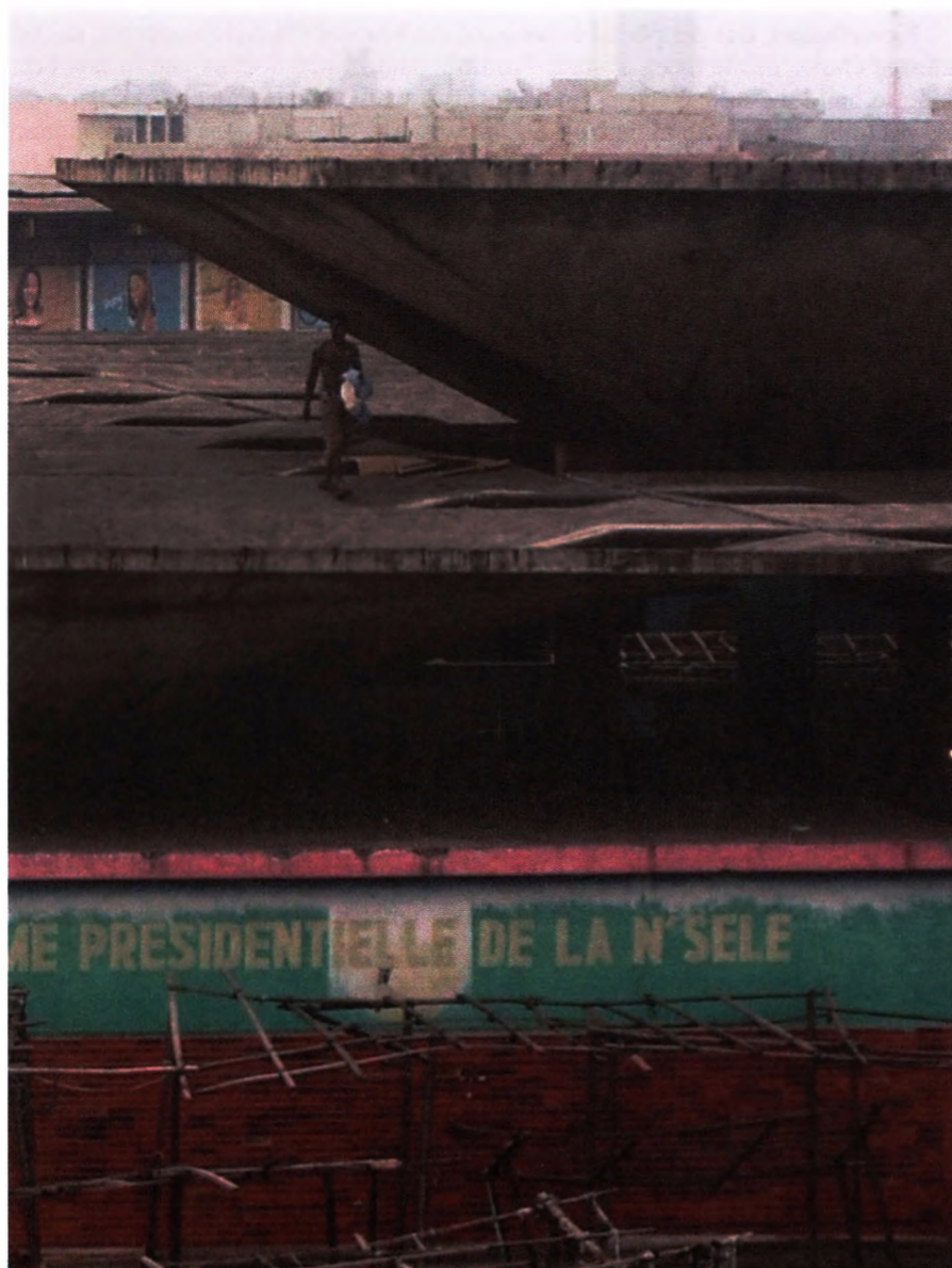
Figure 7: Kinshasa, central market (photograph: Luce Beeckmans, 2008)
