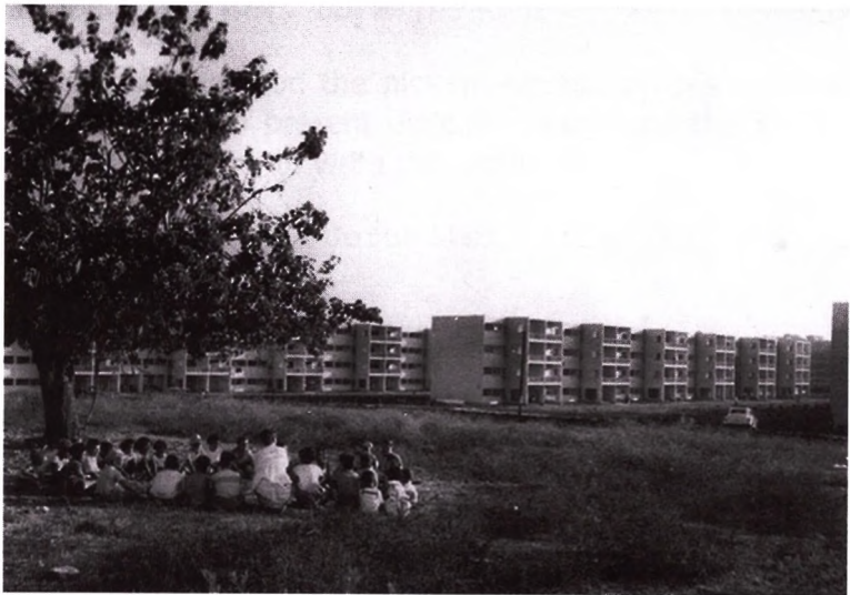
Housing in the Israeli project
