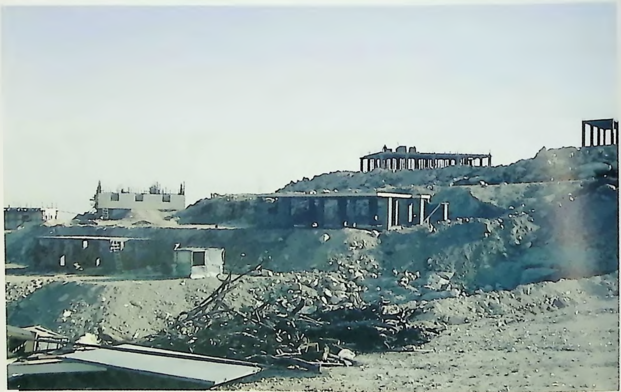
Figure 3 – Beginning of construction
